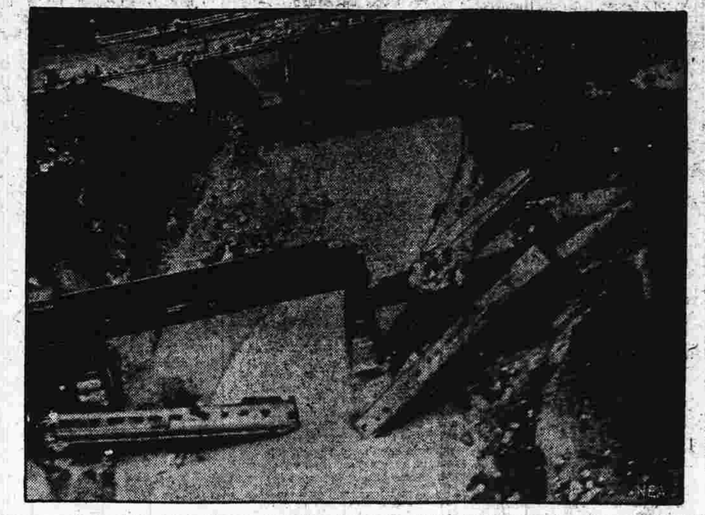
Wreckage of the Golden State Limited, crack Los Angeles-to-Chicago passenger train, which carried eight persons to death and more than 40 others to serious injury when it plunged off a good-weakened bridge near Tucuman, N. M., is pictured above. This photo was taken from an airplane a short time after the disaster.
